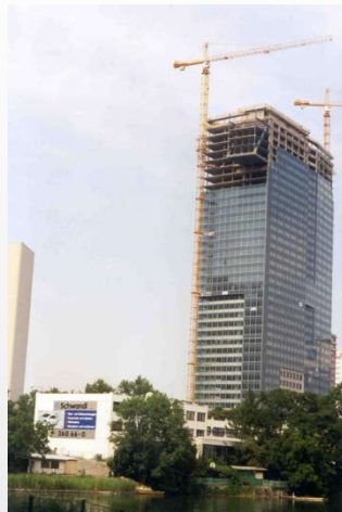
IZD Tower Steel-construction „Hammerkopf“ built 2000
